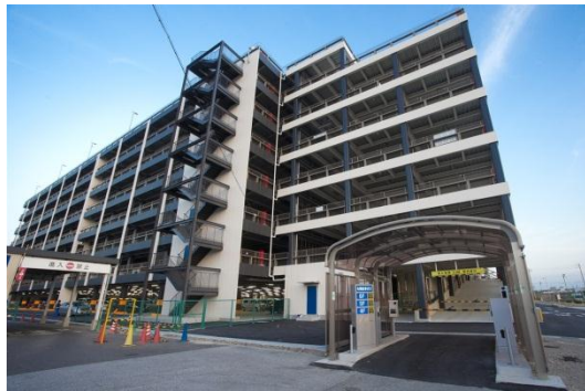
Multi-level stock yard
