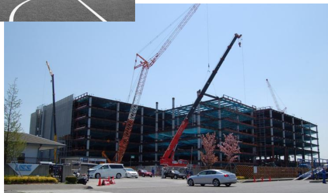
Construction site of USS Nagoya
